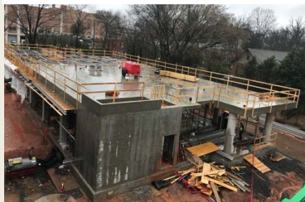
Part I Podium Stripping
