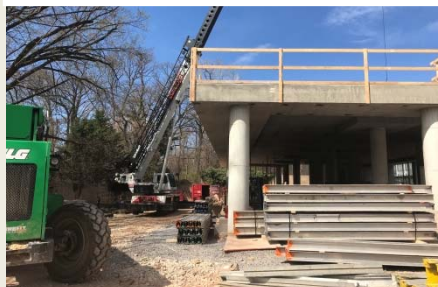
Crane mobilized on site
