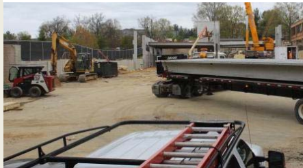
New Pre-Cast Delivery & installation
