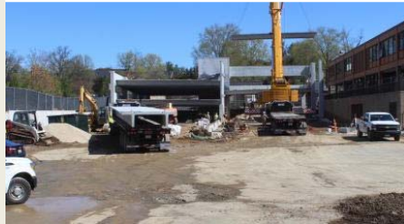
Installation of New Pre-cast
