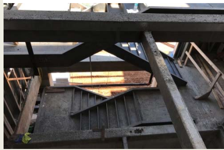
Metal Pan Stair installation
