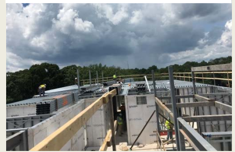
Roof slab prep
