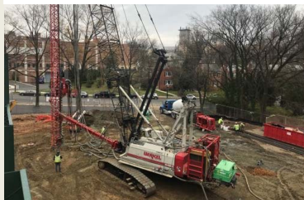
Drilling in Progress
