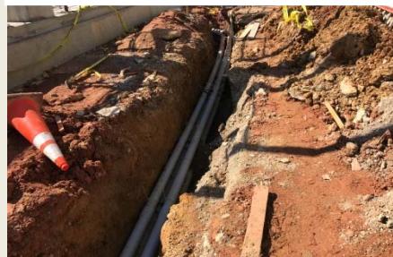
Subgrade Tele-Com Installation
