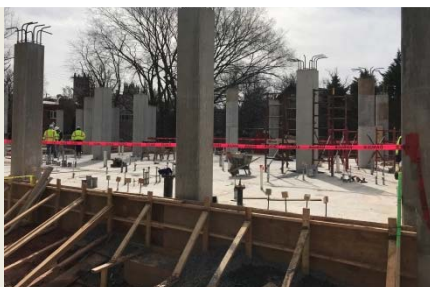
Slab on grade Part 1
