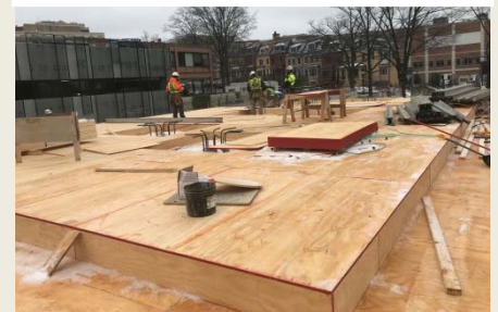
Podium Slab Preparation
